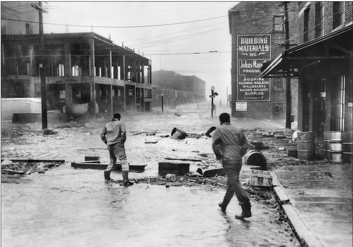
STORM DAMAGE: Water stood waist-deep in this 1954 photo taken at the height of Hurricane Carol, at the intersection of Union and North Front streets in New Bedford. The receding tide left streets littered with downed power lines and shattered property. (Courtesy of Spinner Publications.)
